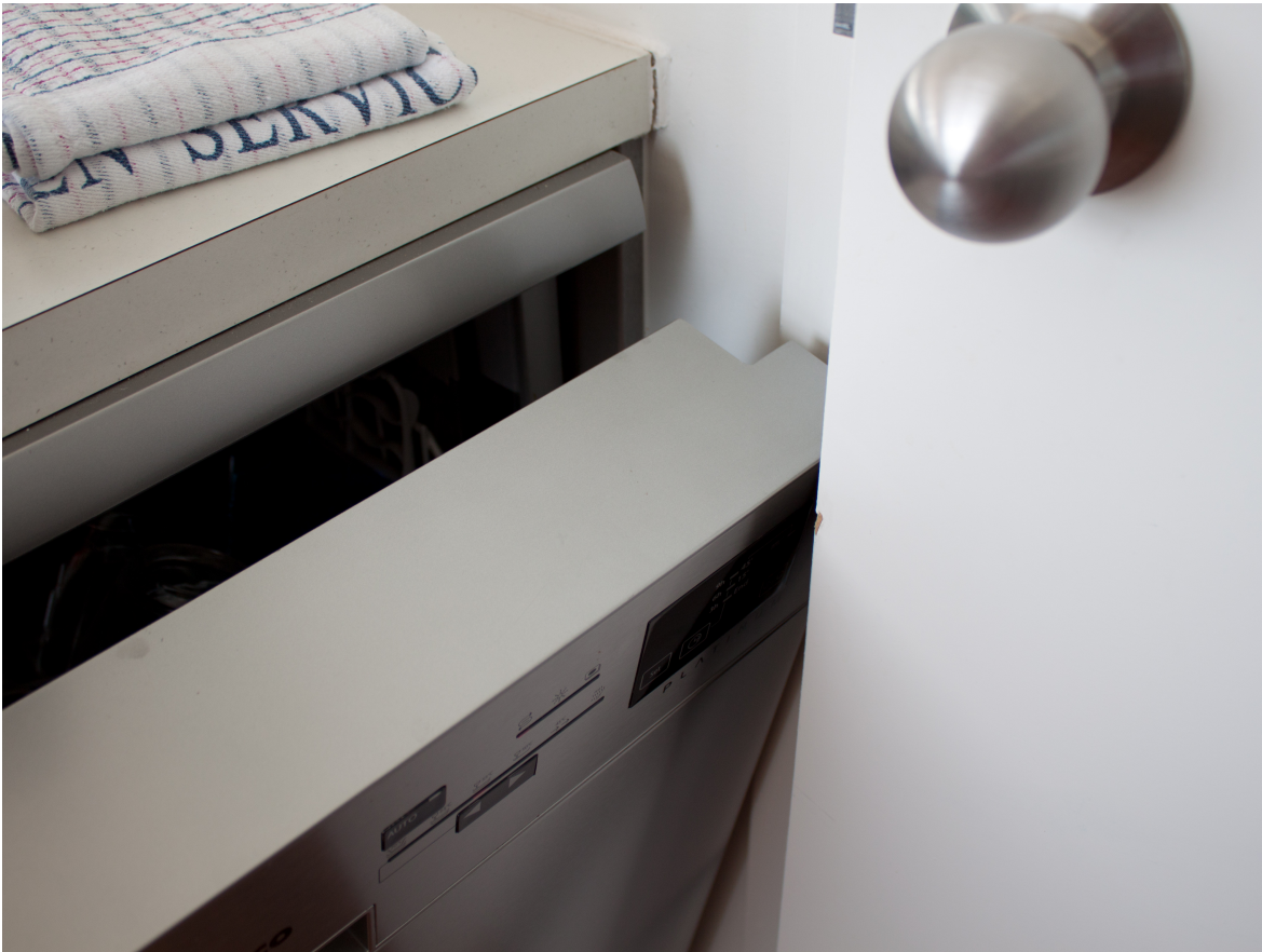
Figure 6.1: A design flaw in a completed kitchen, where the dishwasher door and pantry door collide. Damage can be seen on the pantry door.
